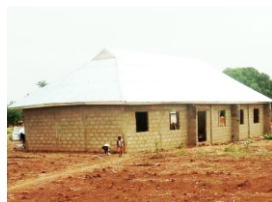
The roof is finally on at Bootinga GHANA
