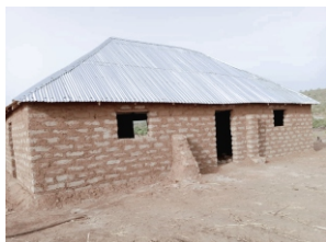
The roof is on at Nanpotibouk GHANA
