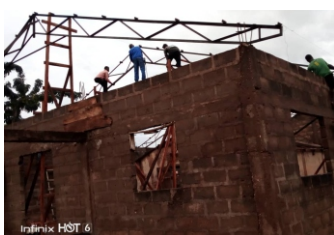
GHANA New roof on Church No. 79
